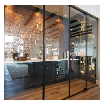
Another consideration for wine room walls is insulated glass units (IGU's). IGU's are made of two pieces of glass with air or gas in between. As discussed previously, these units provide much better insulating factors than a single panel of glass.
